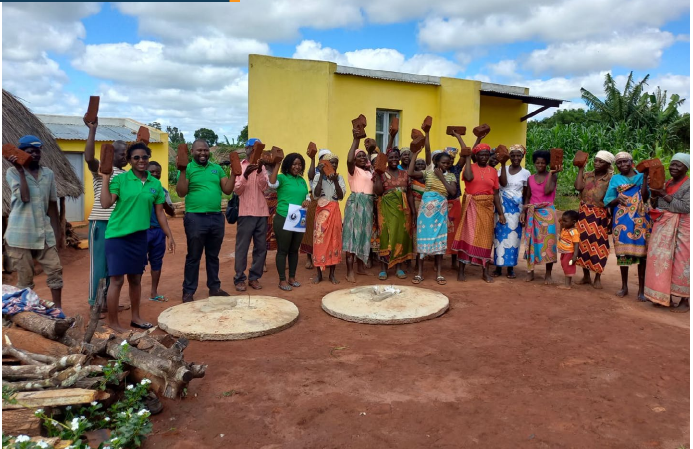
Construction of latrines in Chianga.
