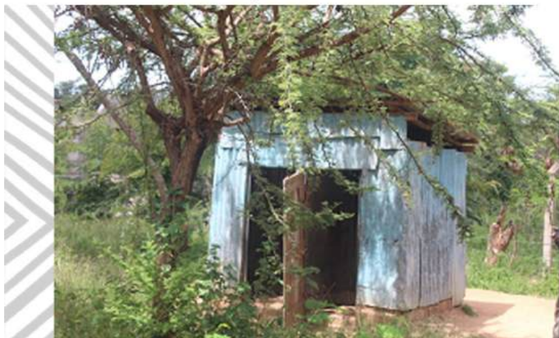
The old washroom facility.
